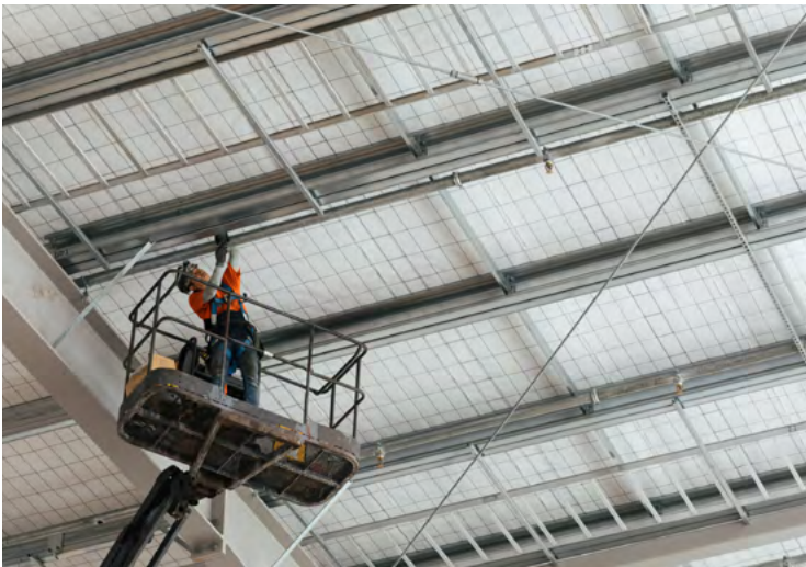
– Roof construction at 30-32 Bowden Road.
